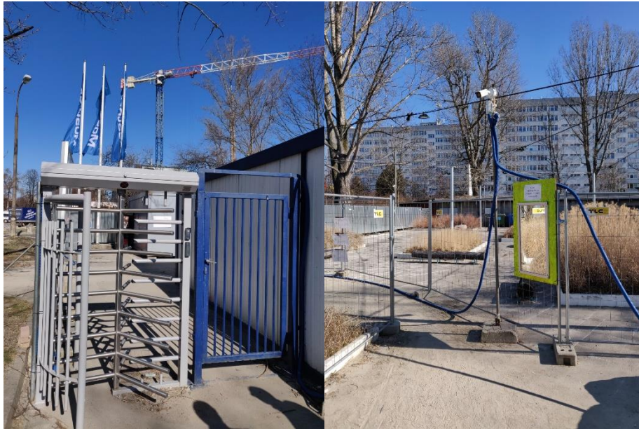
Figure 40. The entrance gates to the office area and the path to the entrance to the construction part.
