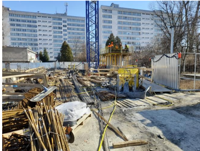
Figure 26: Workers within the construction area
