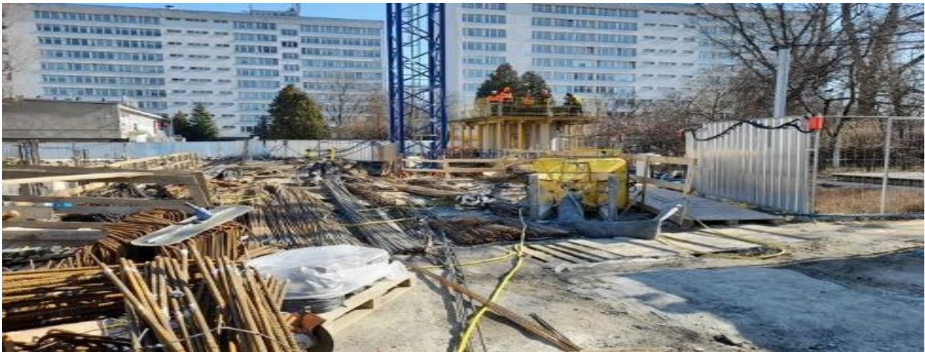
Figure 45. An out-door area in the Pilot site, in which the HSO inspector will perform an on-site inspection using the MR device.
